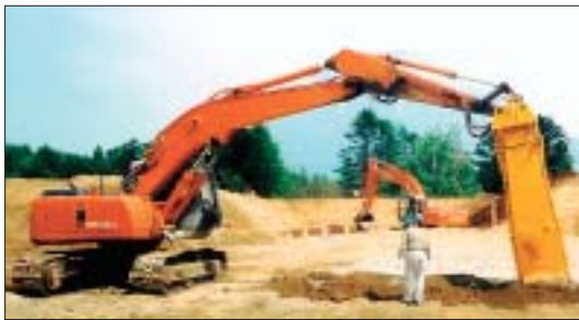
Powder Mixing to reinforce subgrade under embankment
