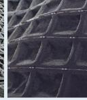
UAV aerial photographic measurement Sample measurement of grating cribs using point group data
