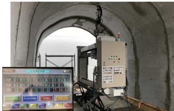
Water-tunnel lining polymer cement mortar spraying system
