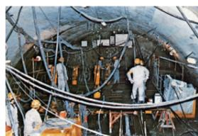
Grouting work in construction of the Joetsu Shinkansen's Nakayama Tunnel
