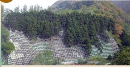
We help to protect communities against slope-related disasters through measures for preventing erosion of artificial slopes due to rainwater, surface water, or other causes, and preventing debris falls, slope failures, and landslides on natural slopes.
