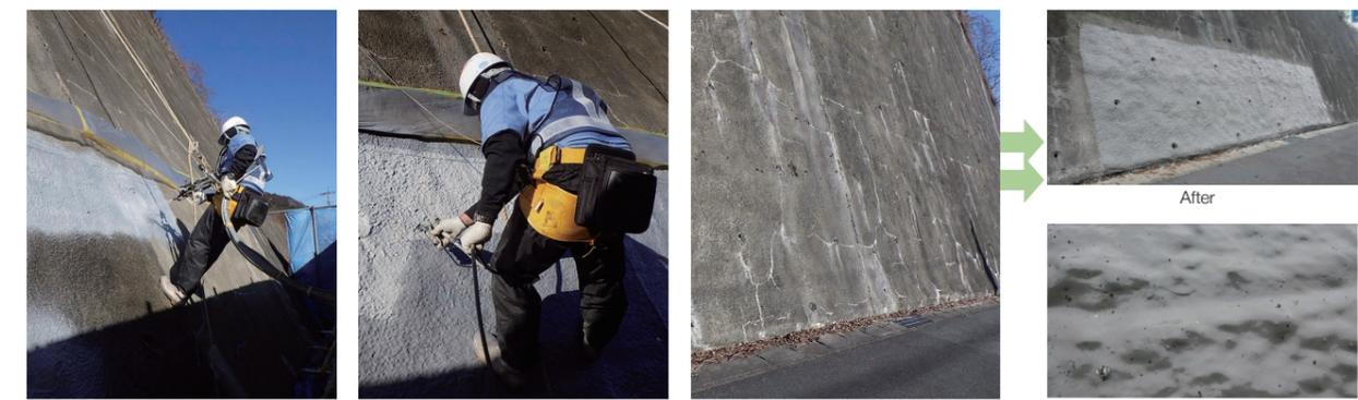
Spraying resin    Spraying the top coat    Before    After (close-up)
