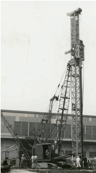
RG pile ground improvement method
