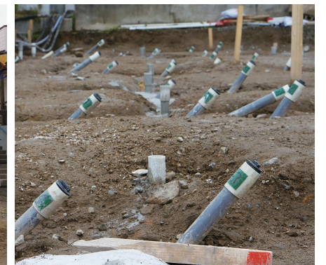
Minimizing building displacement and deformation through permeation grouting
