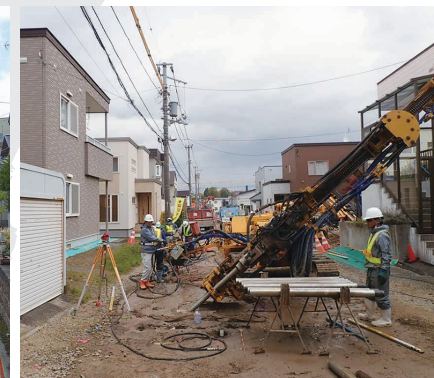
Ground improvement in the lower portion of a residence, using the infiltration solidification processing method
