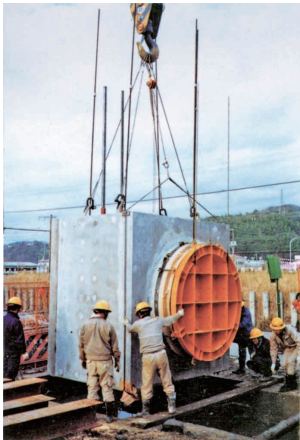
PLUS construction in Yokosuka The "pipe laying under special slurry" (PLUS) method used in pipe construction also was adopted through the technical alliance with Soletanche
