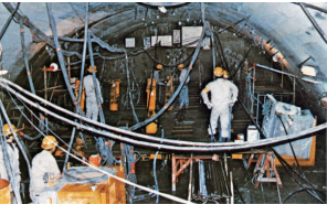
Grouting work in construction of the Joetsu Shinkansen's Nakayama Tunnel
