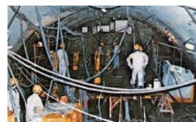
Grouting work in construction of the Joetsu Shinkansen's Nakayama Tunnel
