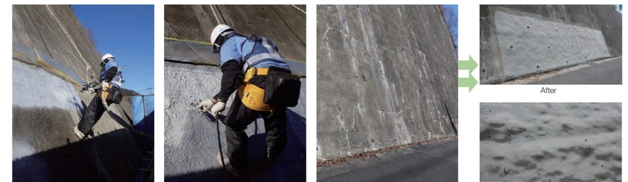
Spraying resin    Spraying the top coat    Before    After    After (close-up)
