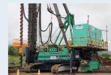
Construction using ICT ground improvement machinery (deep mixing work)
