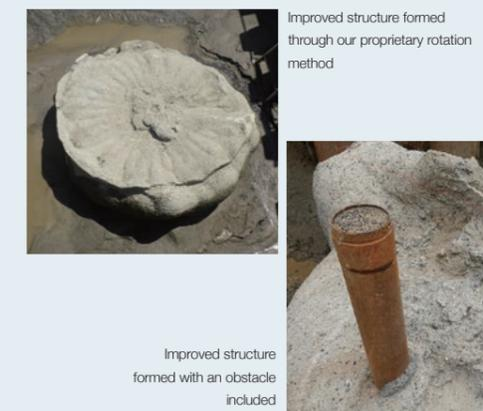
Improved structure formed with an obstacle included
