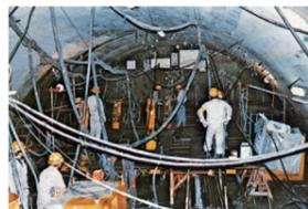
Grouting work in construction of the Joetsu Shinkansen's Nakayama Tunnel
