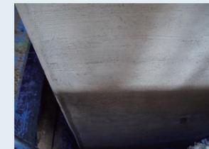
A finished polymer cement mortar surface
