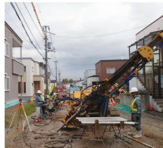
Ground improvement in the lower portion of a residence, using the infiltration solidification processing method
