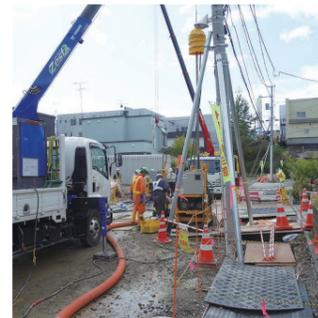
Prevention of liquefaction using the MegaJET method
