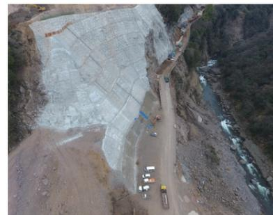
Raito Kogyo was in charge of restoration work on the Choyo Ohashi Bridge Route, including the slopes at Aso Choyo Ohashi and Toshita Ohashi bridges (photo), which had suffered surface collapse.
