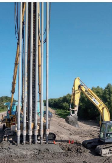
Mississippi River (U.S.) west bank levee repair and reinforcement (ground improvement)
