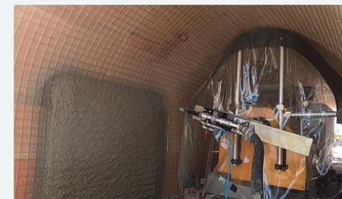
Aqueduct tunnel (existing hydroelectric power generation equipment) lining system
