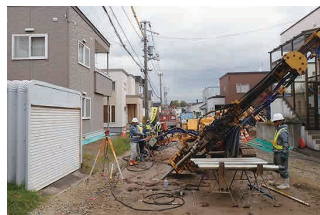
Ground improvement in the lower portion of a residence, using the infiltration solidification processing method
