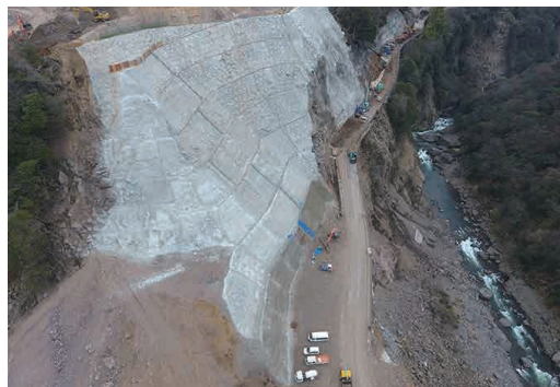
Raito Kogyo was in charge of restoration work on the Choyo Ohashi Bridge Route, including the slopes at Aso Choyo Ohashi and Toshita Ohashi bridges (photo), which had suffered surface collapse.
