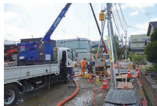
Prevention of liquefaction using the MegaJET method
