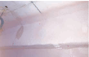
Spray hardened urethane foam
