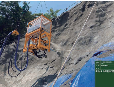
Robo-Shot Type-G mortar spraying
