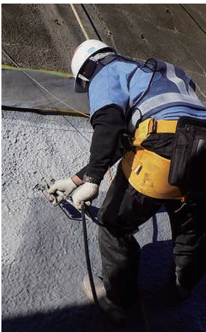
Spraying the top coat
