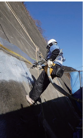
Spraying resin
