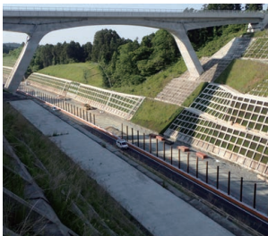
2015 Sanriku Expressway FF slope surface protection work
