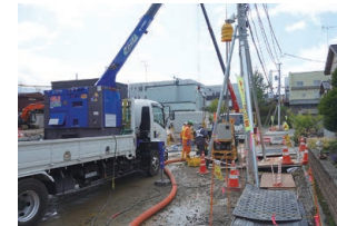
Prevention of liquefaction using the MegaJET method
