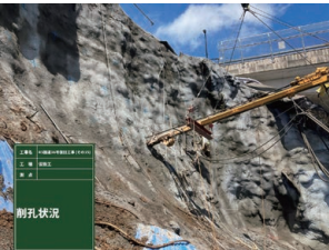
Rock bolt work using suspended Sky Drills
