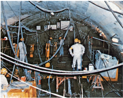
1974 Injection work in construction of the Joetsu Shinkansen's Nakayama Tunnel
