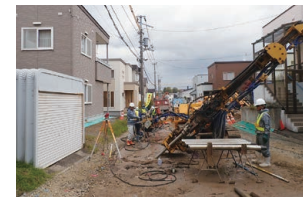
Ground improvement in the lower portion of a residence, using the infiltration solidification processing method
