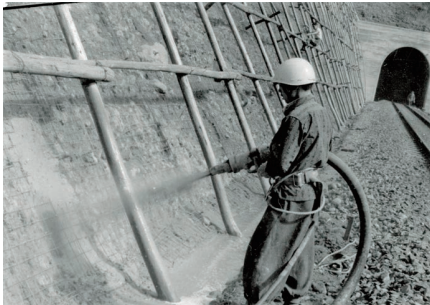
1950 Slope spraying work
