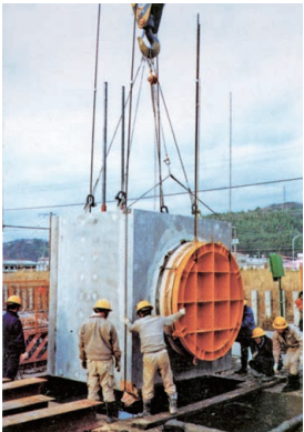
1980 "Pipe laying under special slurry" (PLUSS) method adopted
