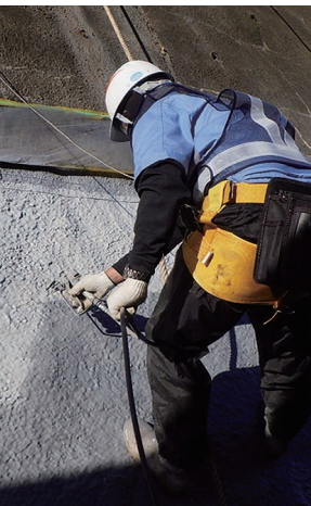
Spraying the top coat
