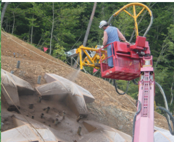
Soil spray works
