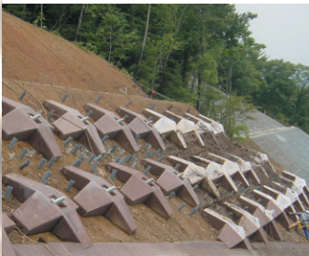
Installed anchor blocks
