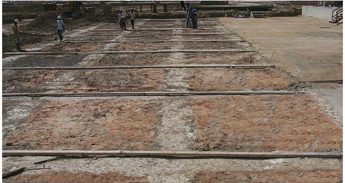
View of CDSM grid prior to construction of mat foundation
