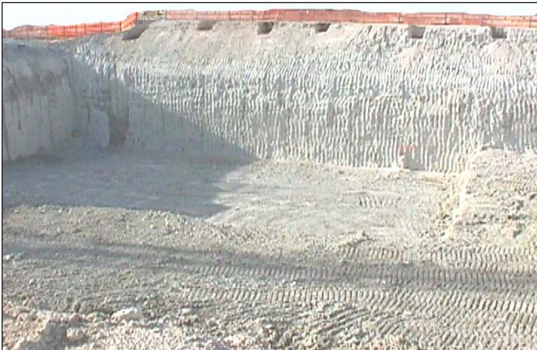
Figure 16: A View of Excavated CDSM Wall and Foundation
