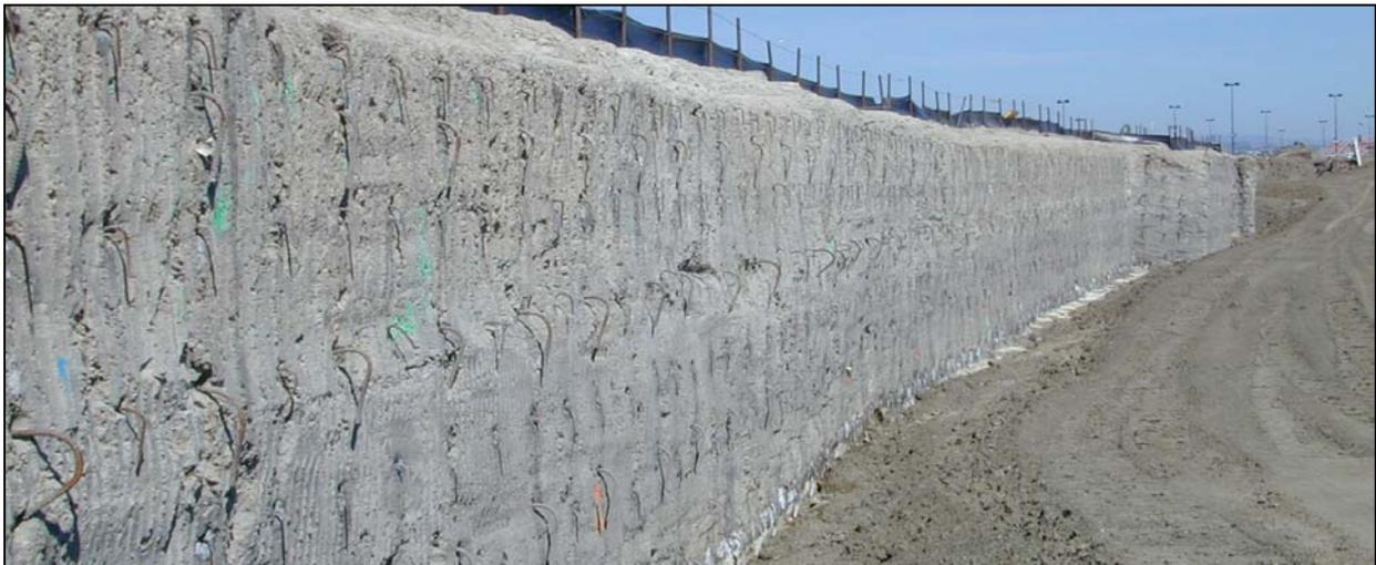
Figure 11b: CDSM Gravity Wall Close-up View of the Left Wall
