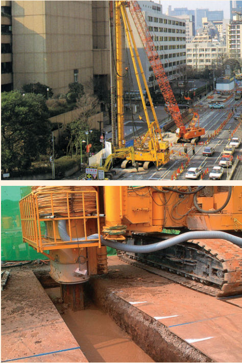
EC Wall installation using RSW
