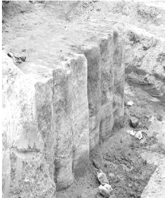
Completed CDSM panel exposed for viewing
