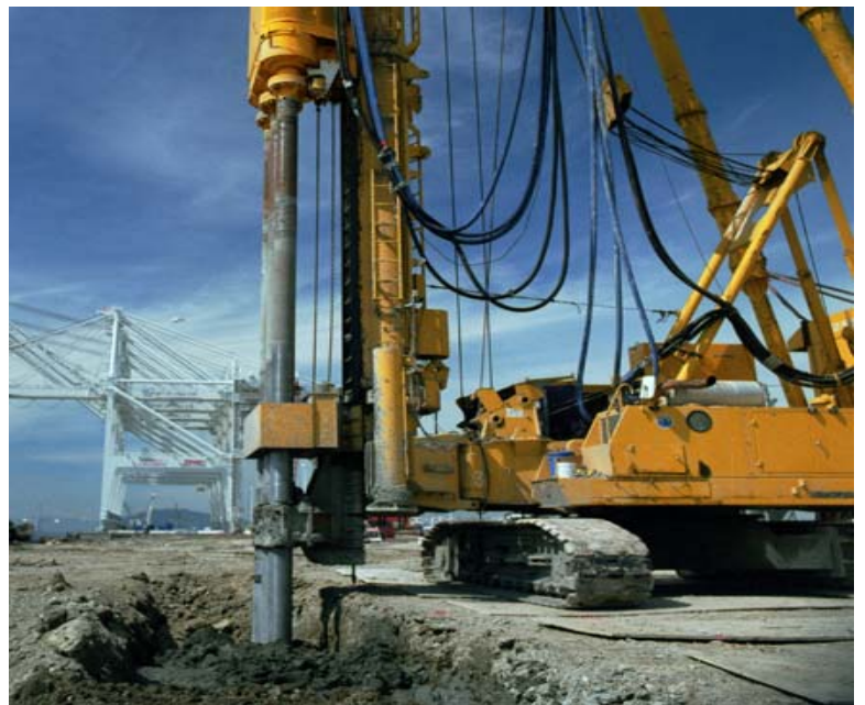
Soil Mixing on Berths 57/58 with 55/56 (cranes) in background
