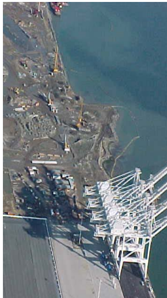
Previous Raito Project (lower right) hosts world's largest cranes
