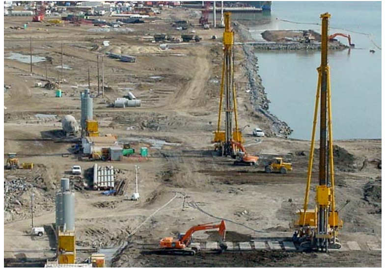
Two Raito Soil-Mixing rigs improving ground for Berths 57/58
