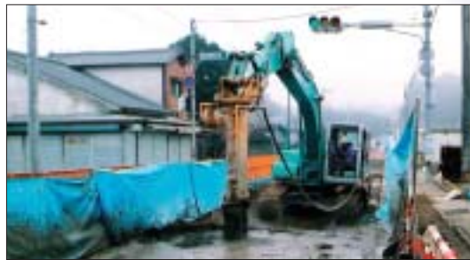
Slurry Mixing to prevent road settlement
