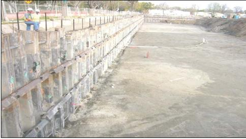
Figure 4: Soil-cement Tied-Back Wall with Sheet Pile Excavation Support System
