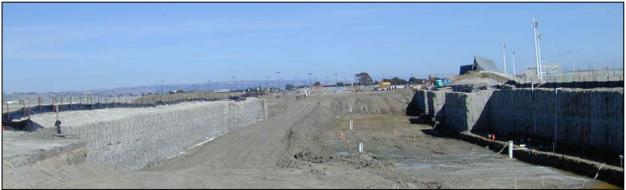
Figure 11a: CDSM Gravity Wall Before Installation of Facing
