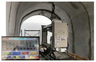
Water-tunnel lining polymer cement mortar spraying system
